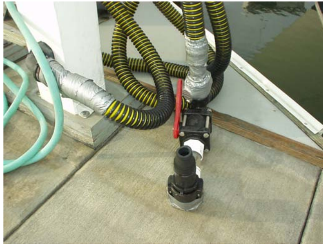
Photo taken 9/10/02. Nozzle duct taped together.
