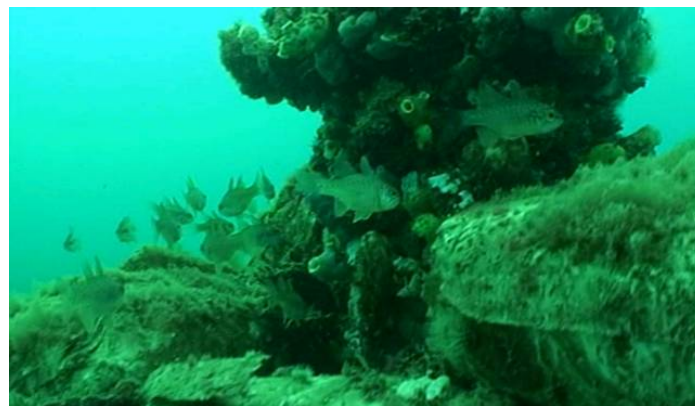
Figure 4: Marine growth around diffuser
