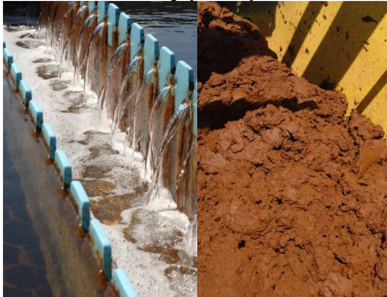
Figure's 9 and 10: 'Densadeg' – settling tank and typical sludge after being put through a centrifuge
