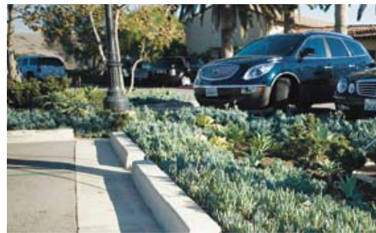
Newport Coast: Slotted curbs allow runoff to flow into parking lot planters, where it can soak into the ground instead of draining to the ocean.
