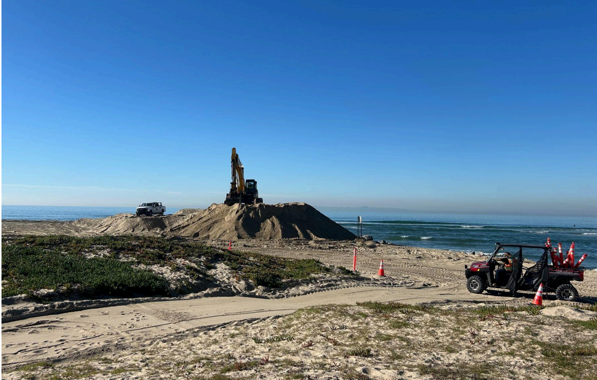
Figure 11. Dredging project ran by county
