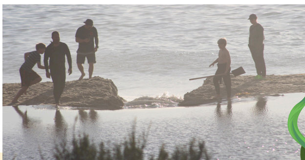
Digging Berm to Surf Creek
